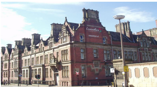
Lancashire County Hall, Preston
